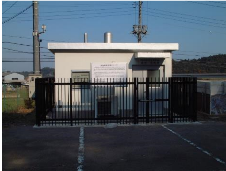
Figure 5.3 Example of installation on a monitoring building (Ibaraki Prefecture)
